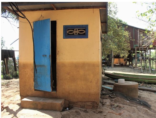
Photo Caption: Latrine shelter in Kampong Thom province with visible flood high water mark about 1.3 meters from ground level.
